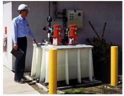
Vertical sump pumps move laboratory wastes from building corner tanks to a collection tank. Lab wastes are blended with other plant process wastes before treatment and discharge.
